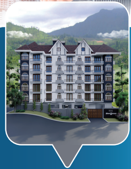
NO. 02 GLENFALL ROAD NUWARAELIYA
